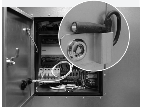
Figure 17 – Box closure with a triangular key
