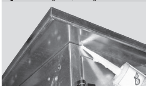
Figure 13 – Sealing of the panel edges
