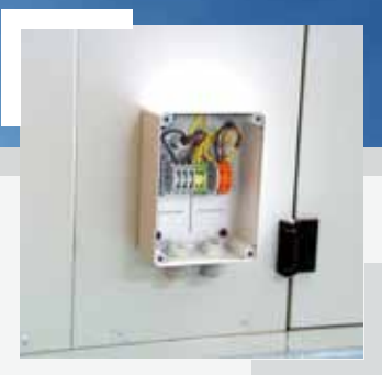
WIRING TAKEN OUT TO WIRING BOXES
